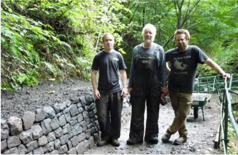
Three dry stone dykes completed. Not only do they enhance the glen, the dykes will help to hold back earth from the paths. Planting on and in the dykes will also help to secure the earth.
