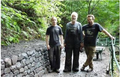
Three dry stane dykes completed. No only do they enhance the glen, the dykes will help to hold back earth from the paths. Planting on and in the dykes will also help to secure the earth.
